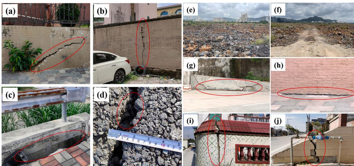
**Fig. 6.** The field investigation photos in Zhuhai. (a-b) Wall cracking phenomenon caused by foundation subsidence in Doumen district; (c-d) pavement cracking phenomenon caused by subgrade subsidence in Jinwan and Xiangzhou districts; (e-f) the reclamation areas near P1; (g-h) the nearby areas of P2; (i-j) the nearby areas of P3.
